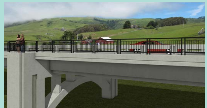
Above: Type 80 bridge rails along the proposed bridge span
